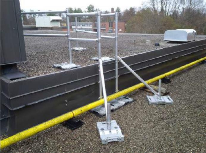
Figure 7: Complete RoofStep System
